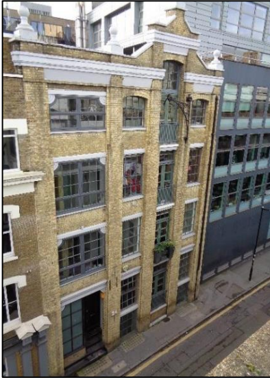
Figure 30: 17-18 Clere Street (western elevation)
