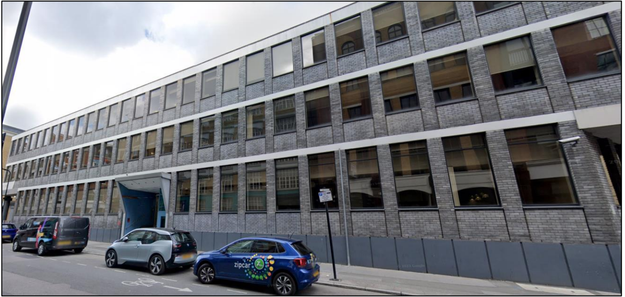
Figure 6: Paul Street elevation, looking south
